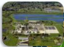
Waste Water Plant
