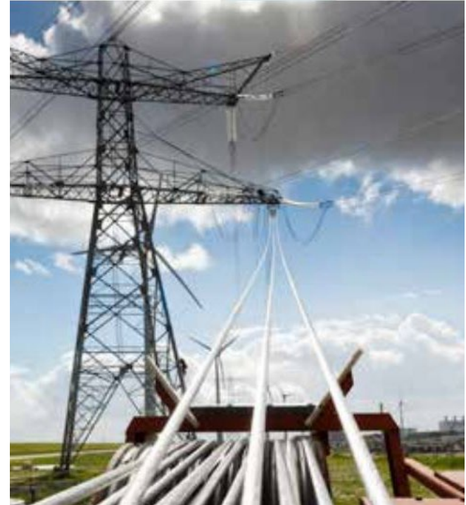
Reconductoring at congestion points To interconnect more offshore wind (Netherlands & Germany)
