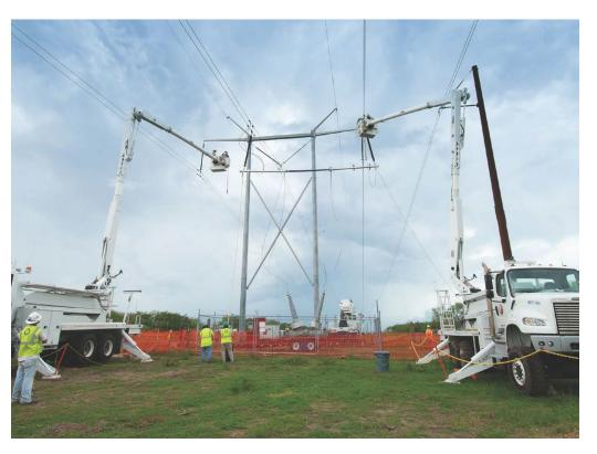
Reconductoring on existing T&D structures with high-efficiency advanced conductor is the fastest, lowest-cost way to add substantial capacity to the existing grid.
